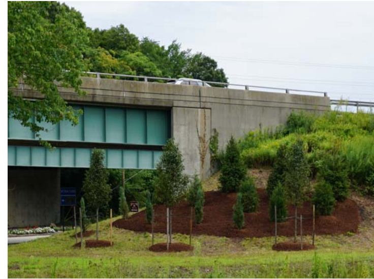
The northwestern slope of the Exit 3 overpass area.
