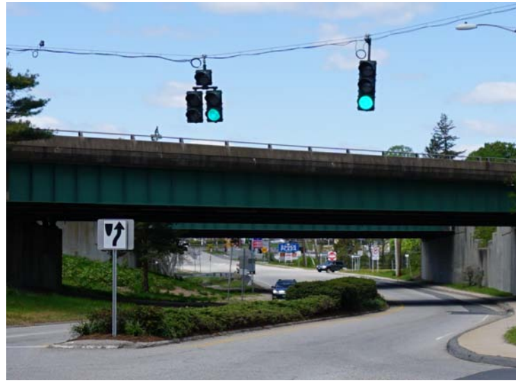
The Route 9, Exit 3 bridge overpass received a fresh coat of paint in April thanks to a collaborative effort.
